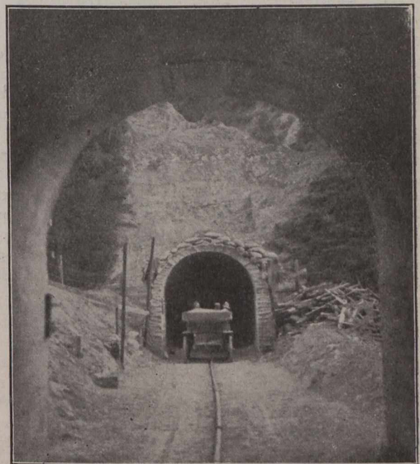
Showing Completed Tunnels.
