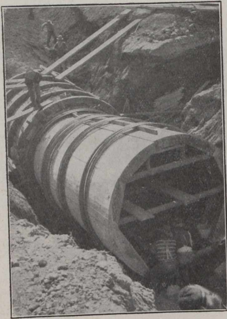
Building a Concrete Siphon.
