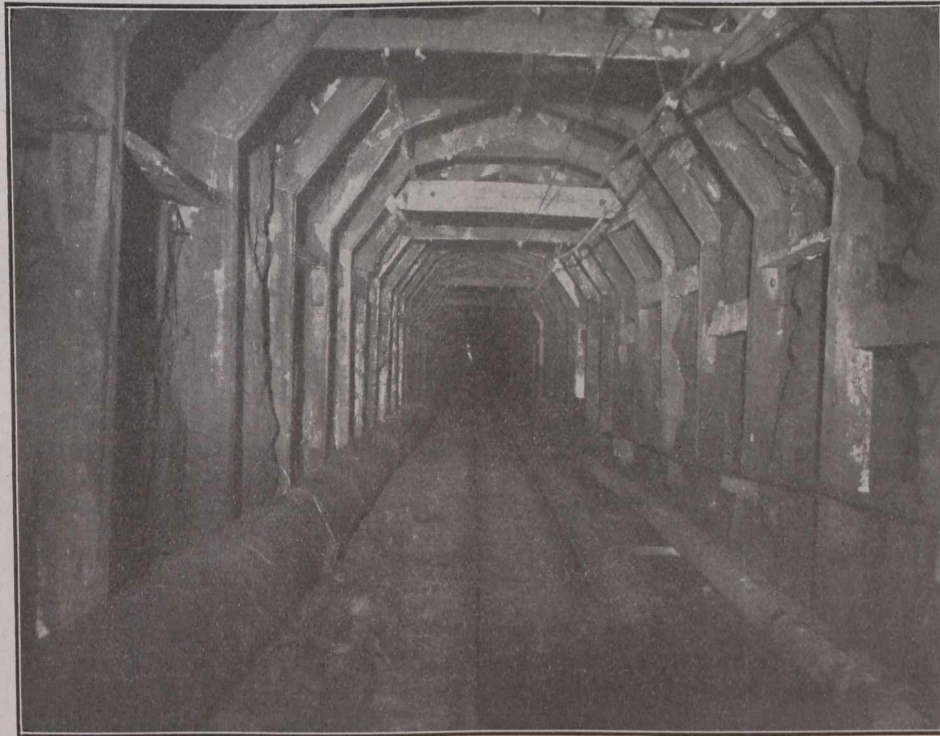
Interior of Elizabeth Tunnel.
