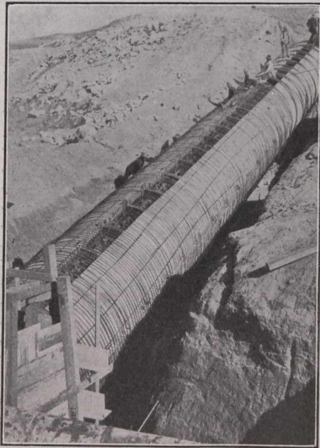
Constructing One of the Concrete Siphons.
