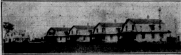
These substantial Workmen's Houses are built by the Miram Walker Co., Walkerville, Ont., using Stucco laid on a foundation of
