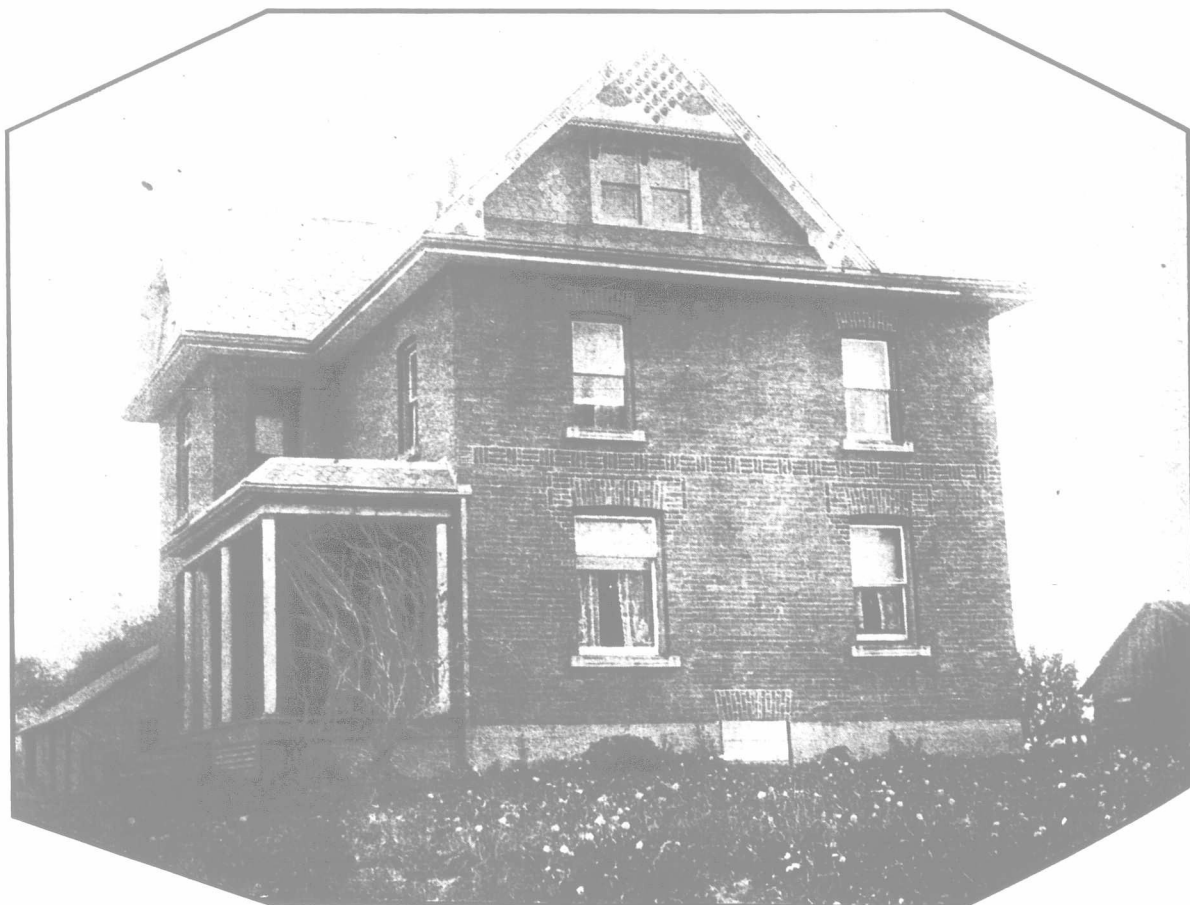
A Substantial Farm House—More Trees Would Improve the Surroundings.
