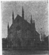
COLBORNE STREET METHODIST CHURCH, BRANTFORD
