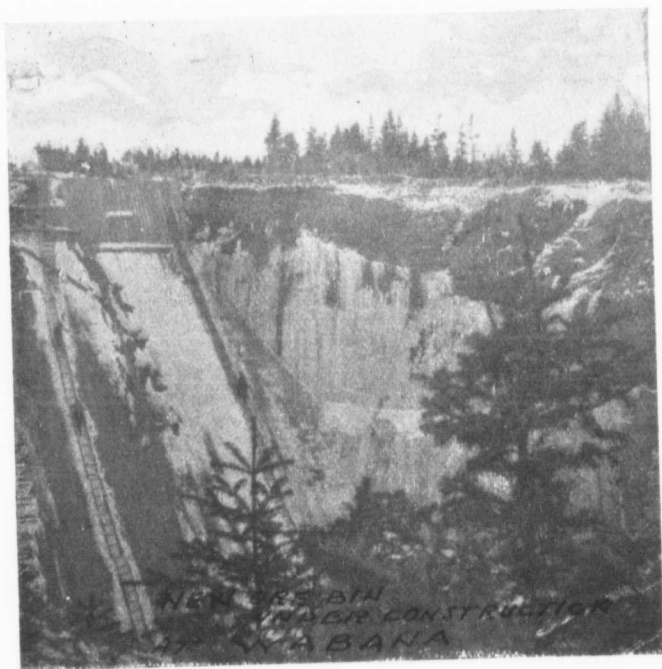
New Ore-bin under construction at Wabana.
