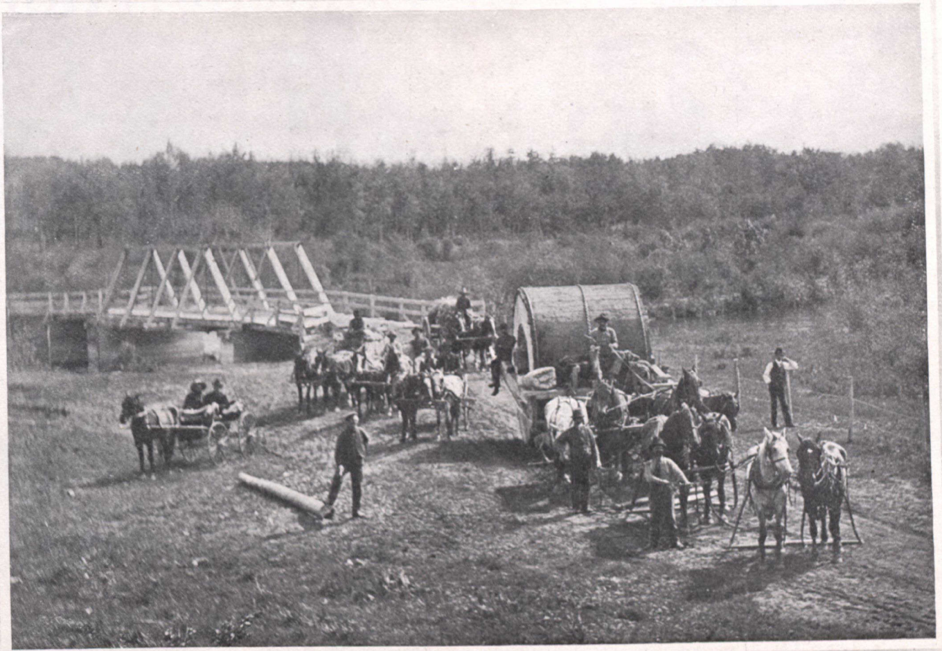
A Marine Boiler made into a "Roller" and "Rolled" a Hundred Miles, from Edmonton to Athabaska Landing.
