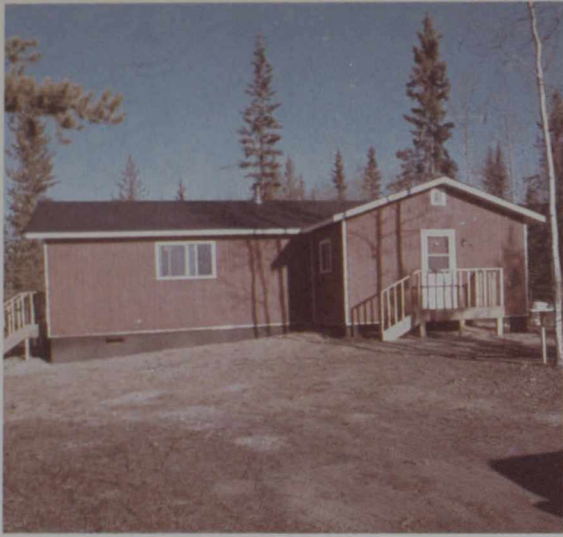
The red house shown here was built by Beavers at Peerless Lake in Northern Alberta, with help from local people, for under $13,000 in materials. It is framed in 2 x 6s. With R20 insulation and a wood-burning heater, it is snug at 40°F below.
