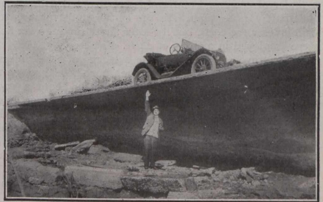
Washout Under a 14-Foot Brick Road in Ohio.
