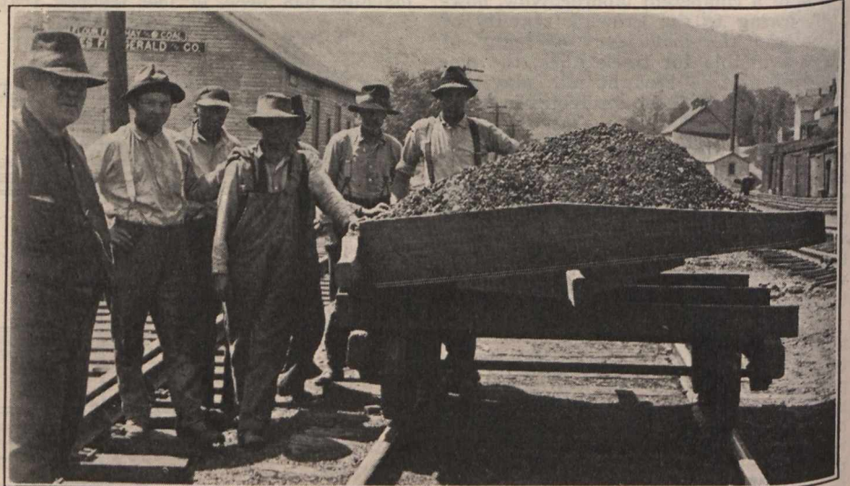
Push car, dump box filled.
