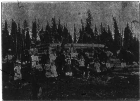
Building a Log House in New Ontario.
