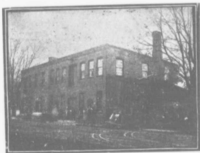
W. H. Carson & Sons' Planing Mill, Oakville.
