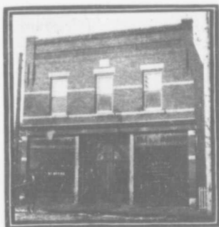
Post Office Block, Oakville
