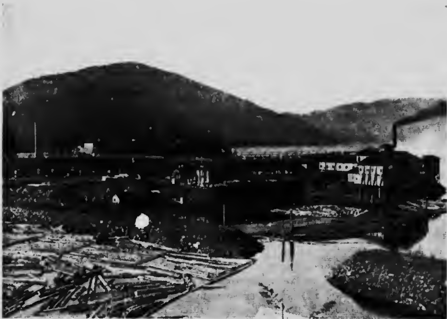
Seal Cove sawmill and Canadian Fish and Cold Storage Company's plant (rear view), Prince Rupert, British Columbia.
