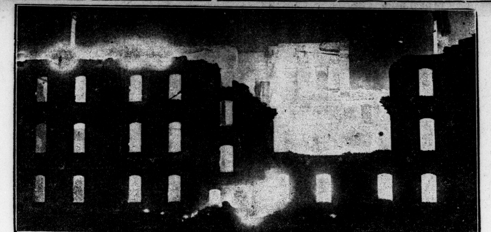
RUINS OF ST. BONIFACE COLLEGE, WHERE TEN LIVES WERE LOST IN THE FIRE WHICH SWEEPED THE COLLEGE ON SATURDAY MORNING. THIS PICTURE WAS TAKEN AT 4 O'CLOCK, AND SHOWS THE SOUTH SIDE OF THE COLLEGE, WHERE THE LABORATORY WAS LOCATED. THE KU KLUX KLAN OR THEIR SYMPATHIZERS ARE SUSPECTED OF THE OUTRAGE BY THE JESUIT FATHERS CONNECTED WITH THE INSTITUTION, WHICH WAS ONE OF THE OLDEST ROMAN CATHOLIC COLLEGES OF CANADA. ST. BONIFACE IS ADJACENT TO WINNIPEG.
