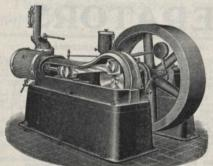
are all fitted with automatic governors and run at regular speed, whether loaded or light.
