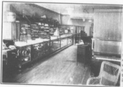
Another interior vision of the new Kellestine Store, Owen Sound
