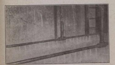
Showing Flush-water Passing Through Apertures in Bottom of Air Supply Crid.
