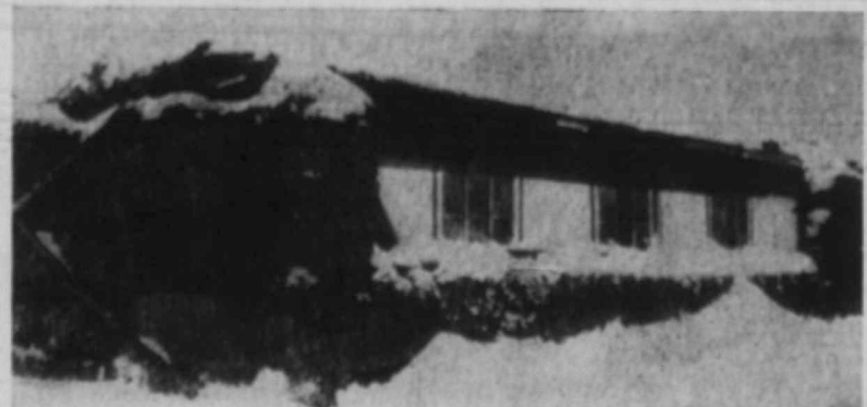
Straw Poultry House Straw is baled and forms three sides of the house and part of its front. It is dry and very satisfactory. A number are in use in various places.
