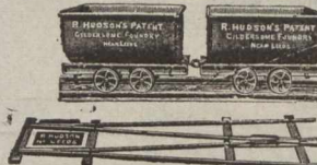
39—Pass-by, with Fixed Points Castings only
