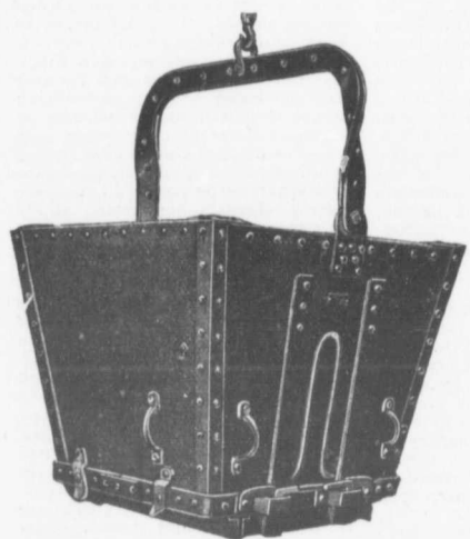
Furnished with either heavy steel drop balls or chains
