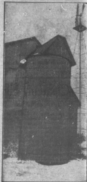
A Stave Silo That Has Been Giving Good Service Since 1893.
