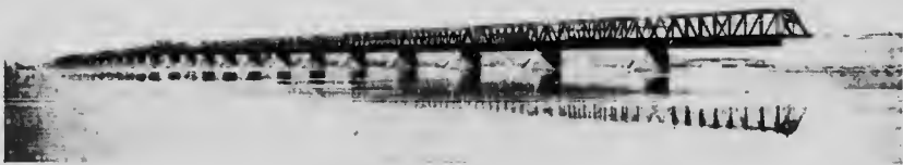
Grand Trunk Victoria Jubilee Bridge over the St. Lawrence River, Montreal.
