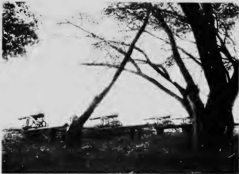
A Glimpse of the Old City Wall and Bailements.
