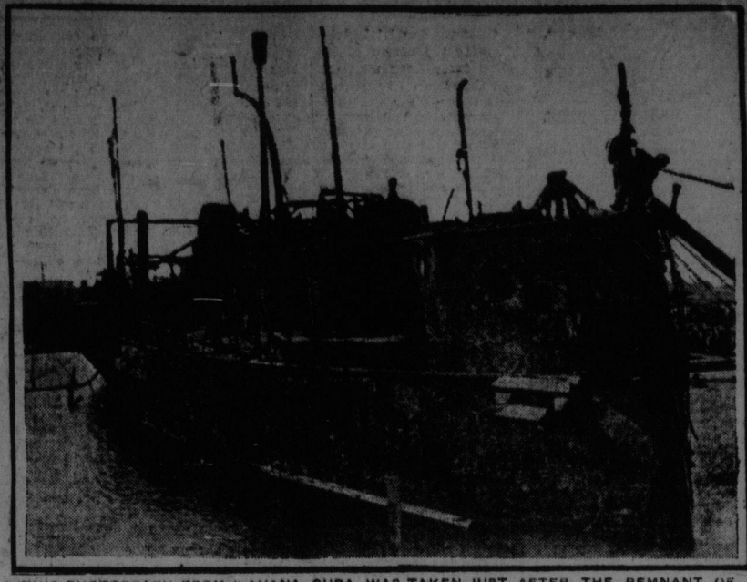
THIS PHOTOGRAPH FROM HAVANA, CUBA, WAS TAKEN JUST AFTER THE REMNANT OF THE BATTLESHIP MAINE WAS FLOATED TO THE SURFACE OF HAVANA HARBOR, BY PUMPING WATER INTO THE TEMPORARY COFFER DAM BUILT ABOUT THE WRECK. THE HULK WILL BE TAKEN OUT TO SEA SOON AND SENT FINALLY TO THE BOTTOM.
