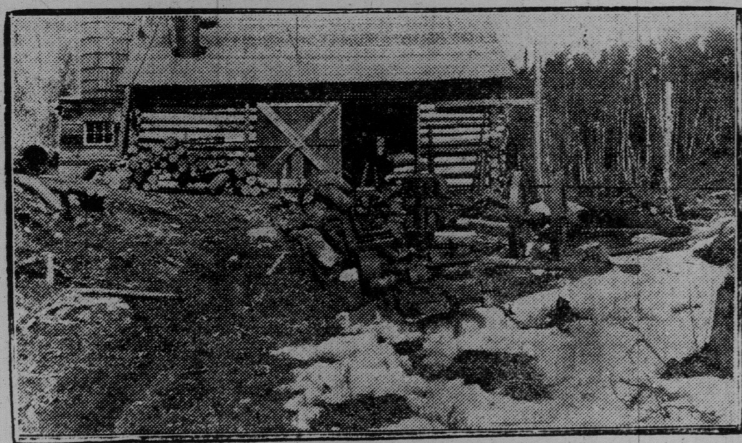
WASAPIKA BOILER HOUSE.
