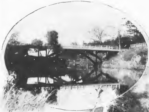
The Gorge Bridge.
