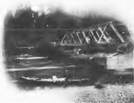
Cowichan River Bridge.
