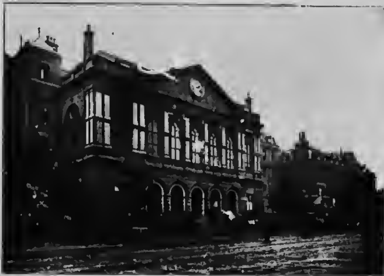
LONDON HOSPITAL, MILE END ROAD.
