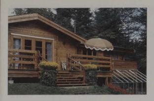
Pan-Abode Buildings of British Columbia sells pre-cut, 3" by 6" and 4" by 6" logs which you can stack up into a handsome, quiet and long-lasting house.
