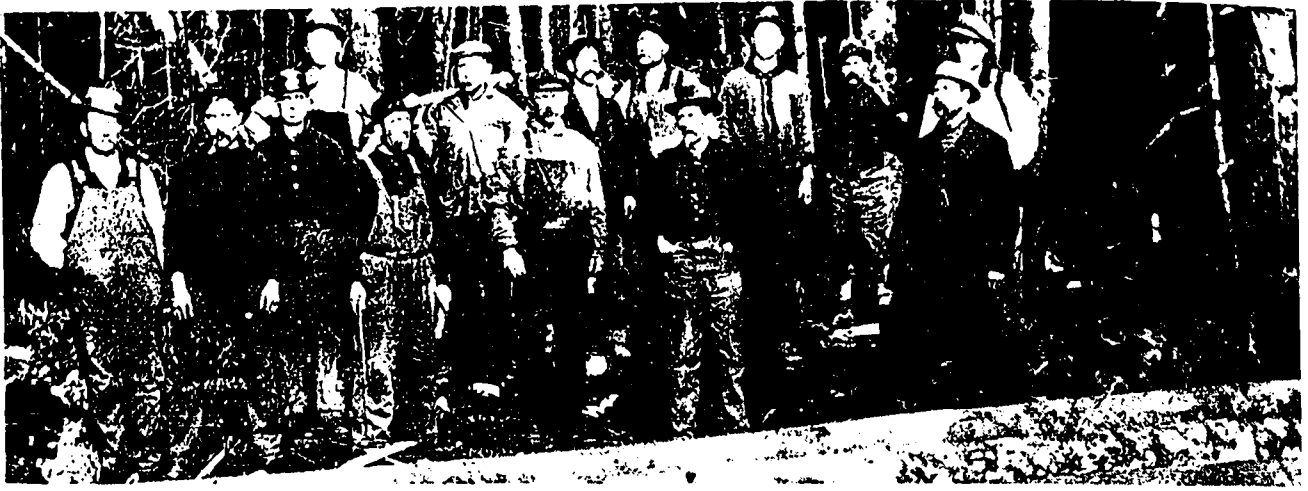
ICELANDERS BUILDING THE FOUNDATION OF THEIR FIRST HOUSE
