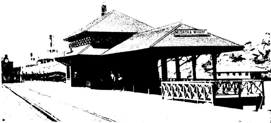
MUSKOKA WHARF STATION.
