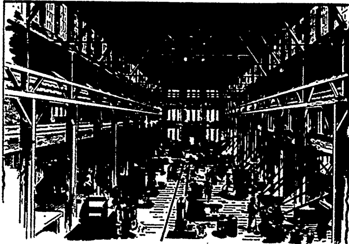
MACHINE SHOP, EDISON WORKS, PETERBOROUGH, ONT.
