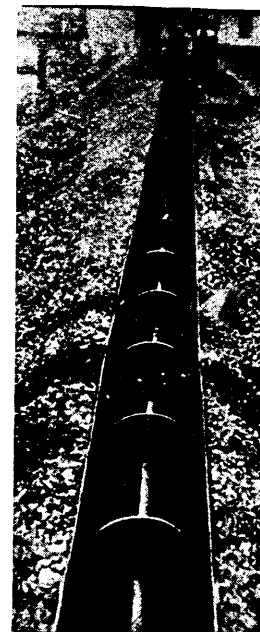
CABLE CONVEYORS FOR HANDLING COAL.
