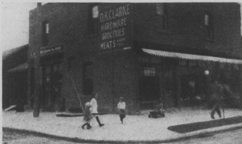
The D. K. Clarke Store, Hamilton, showing the grocery and meat departments in the front and hardware department at the side.
