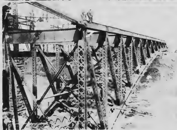
West end anchor bars. West arm cantilevered.
