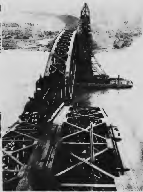
10th 498 foot span ready to launch
