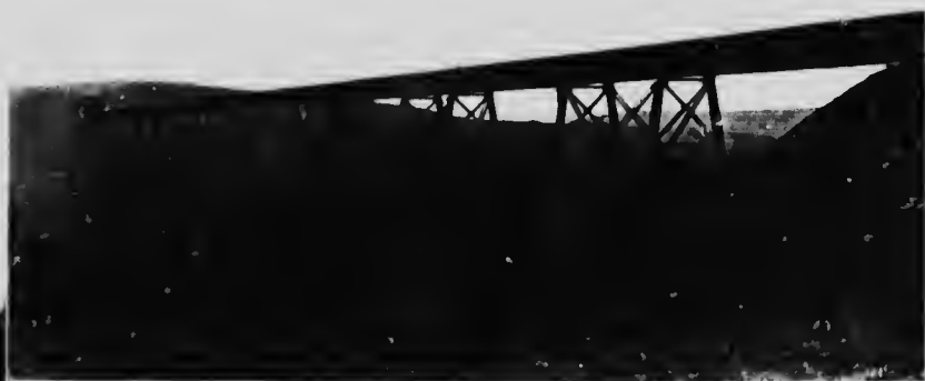
LITTLE SALMON RIVER VIADUCT
