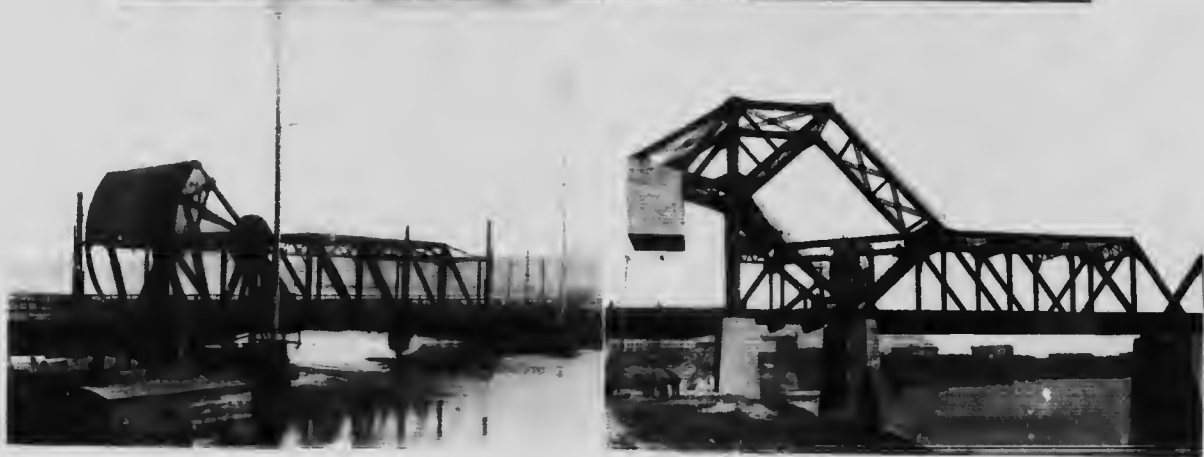
Dorchester Bridge, St. Charles River, Quebec, Gran. St., Vancouver.
