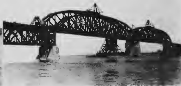
Finishing 1st 108 feet span. Launching 4th 108 feet span.
