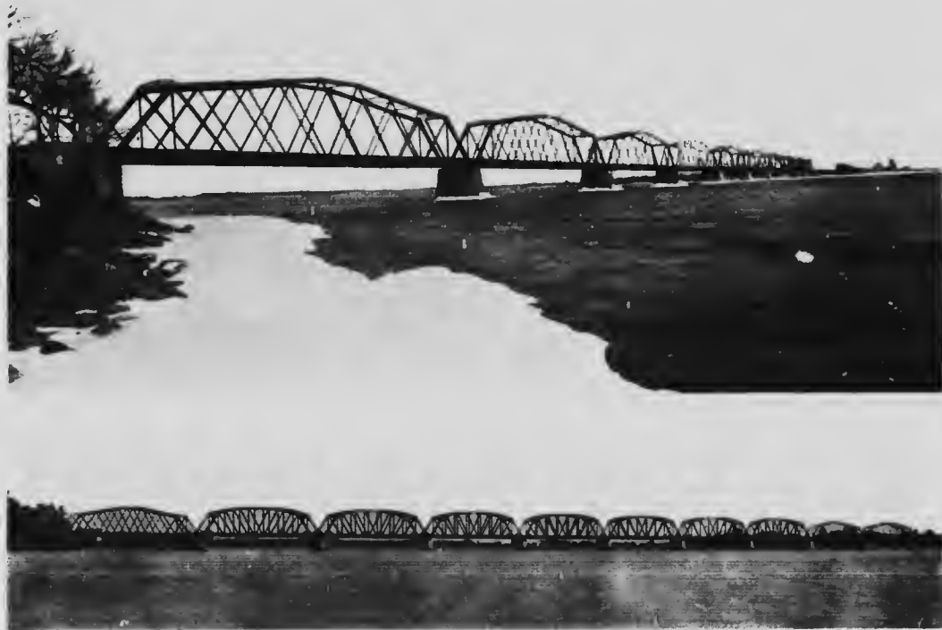
Middle channel spans 1889. Middle channel spans being replaced 1910.
