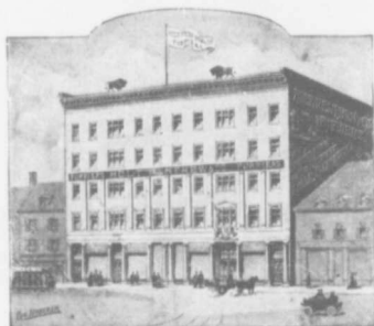
Building of Holt, Renfrew & Co By Royal Appointment, Furriers to the Queen, and Royal Family
