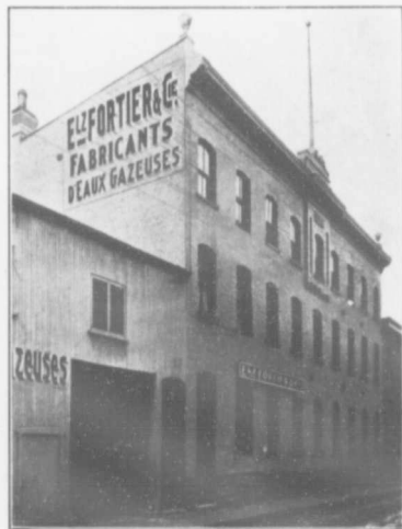
ELSEAR FORTIER & CO. Imposing Brick Structure, 321-323 St. Dominique St. Manufacturers of Aerated Waters.
