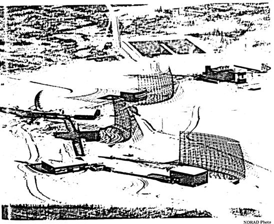
Radar antennas at one of the outposts in NORAD's Ballistic Missile Early WarningSystem cast shadows across the Alaskan landscape. These devices throw long radar beams 3,000 miles or more to spot an intercontinental ballistic missile strike
