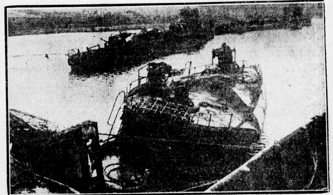
Salvaging operations being undertaken by Great Britain to raise the sunken German fleet at Scapa Flow are shown in the above photograph. The value of the fleet lies chiefly in the enormous mass of machinery and brass and copper tubing it contains
