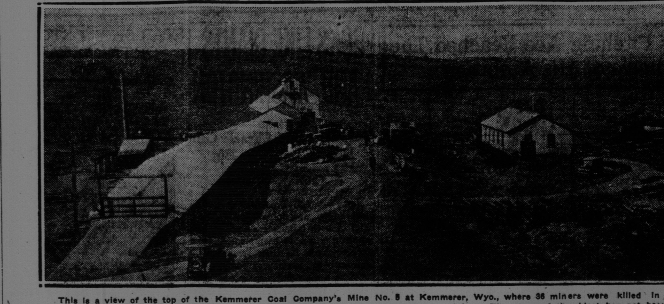
This is a view of the top of the Kemmerer Coal Company's Mine No. 8 at Kemmerer, Wyo., where 36 miners were killed in an explosion. Twelve others entombed at the bottom of the shaft were brought out alive by rescue parties. The cause of the blast has not been ascertained.
