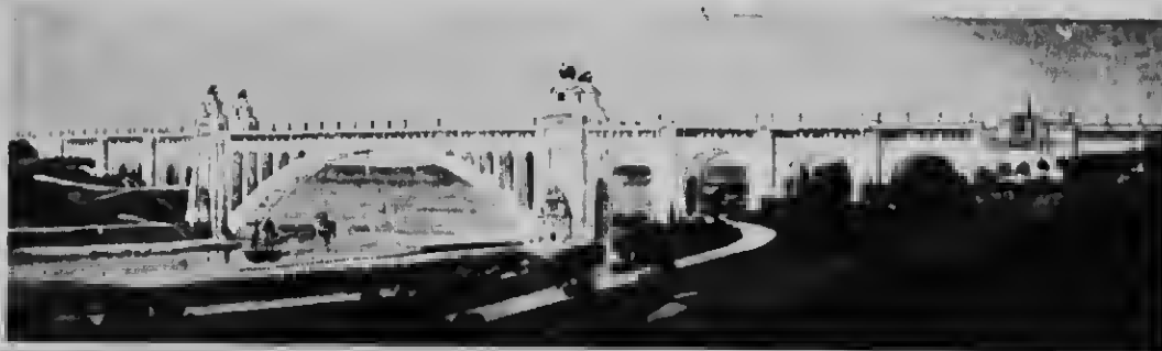
Perspective view of proposed Henry Hudson Memorial Concrete Arch Bridge, as it will appear when completed. It will have a single arch open 703 feet in the clear and a rise of 177 feet centre to centre, or approximately three times as long as the longest Concrete Arch Bridge now in existence.
