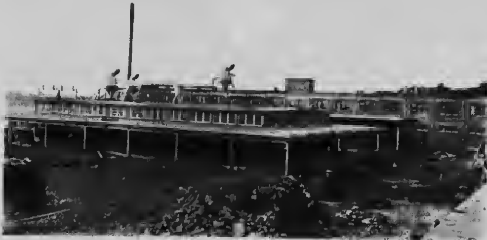
Partial View W. C. Edwards' Mills, Ottawa.
