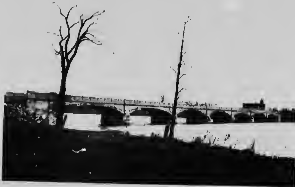
Washburn's Bridge, Ottawa.
