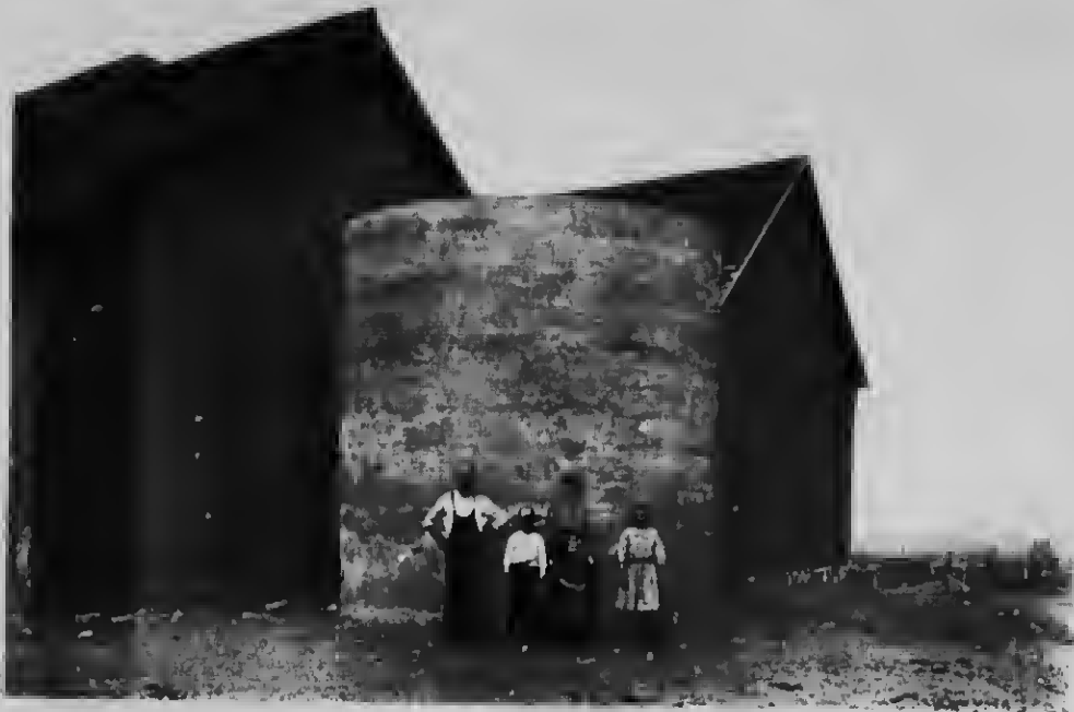
Silo on farm of Samuel Johnston. This silo was built by Mr. Johnston himself in five days. International Portland Cement used.
