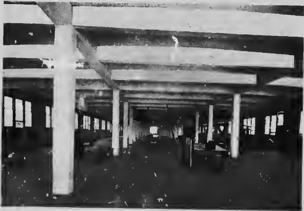
Interior, W. C. Edwards' Mills, Ottawa.
