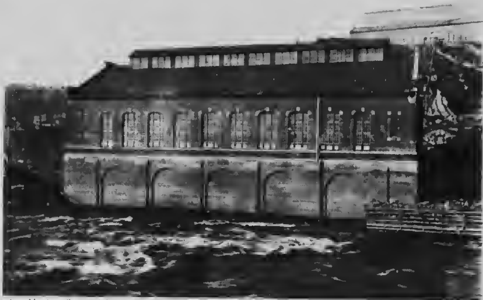
Northern Aluminum Company's Power Plant, Shawinigan Falls P.Q. Over 10,000 barrels International Portland Cement used in building this plant.
