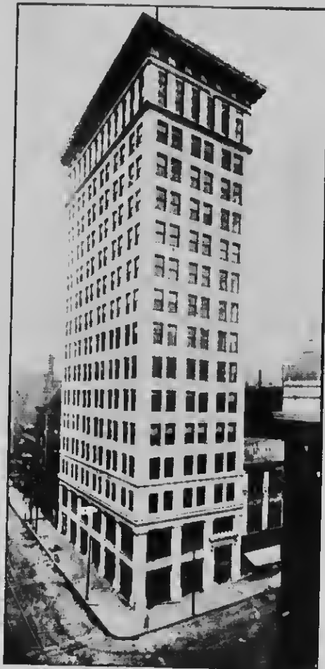
Ingalls Building, Cincinnati. Built entirely of Portland Cement.
