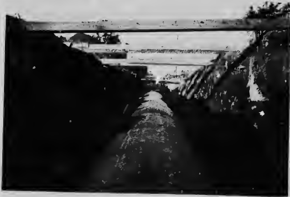
Aqueduct, Montreal Water Works. Length about six miles. Capacity about 60 million gallons per hour. Approximately 50,000 barrels of International Portland Cement used.
