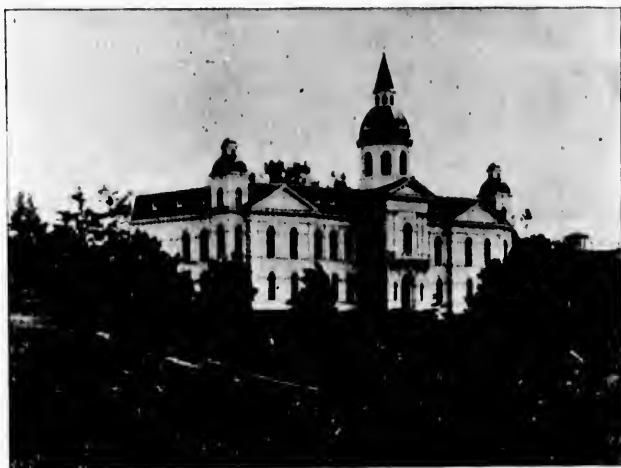
The Main Building of Acadia College, Wolfville.
