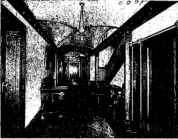
Main Hall, Looking Toward Entrance.
