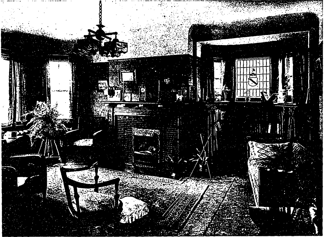
Library, Residence of F. L. Ratcliff, Crescent Road, Toronto. The High Bay Window with its Fixed Shelves Below is an Appropriately Devised Feature. Burke, Horwood and White, Architects.
