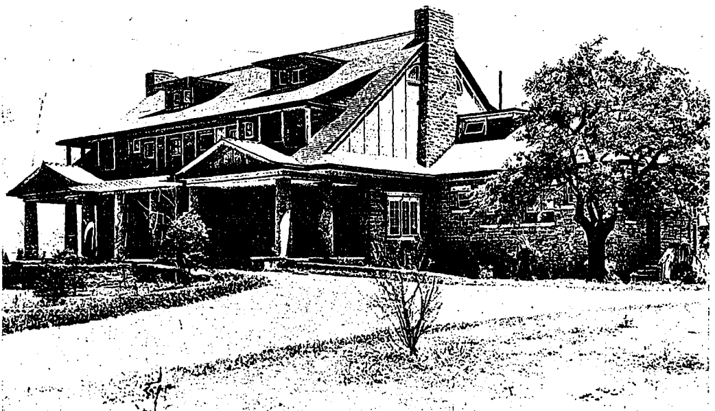
View Showing Service Wing, Residence of A. B. Ormsby, Mimico, Ont. The Walls of this House are of White Limestone, with Cement Stucco Gables, the Pillars of the verandah being of Concrete. F. H. Herbert, Architect.
