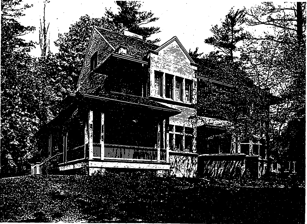
Residence of C. Cambie, 34 Poplar Plains Road, Toronto. The Interest in this House Lies in the Projecting Eaves, Which Give a Sense of Security, and the Spacious Verandahs, Which Suggest Comfort. These Pleasing Features are Accentuated by the Mass of Trees and Foliage in the Background. Bond and Smith, Architects.
