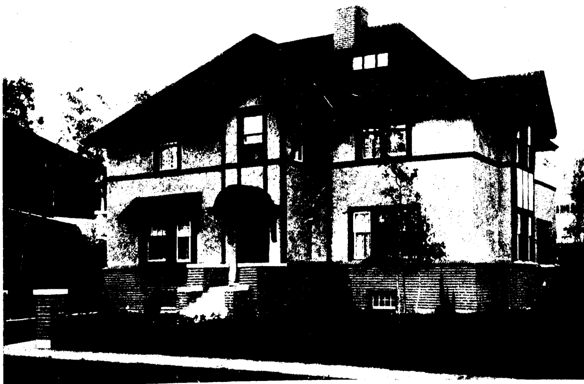
Residence of Mr. F. Christie, Winnipeg. J. D. Atchison, Architect. Herringbone Metal Lath used in these outside walls.
