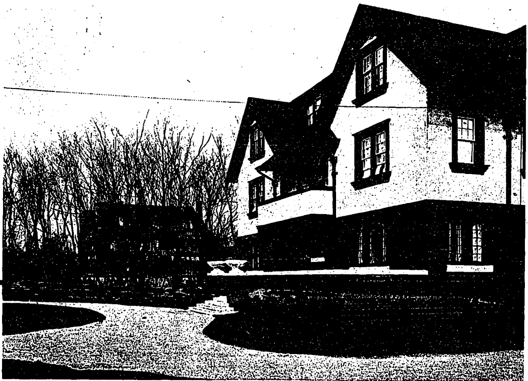
Residence of Hugh F. Osler, Winnipeg. The walls of this Residence are Built of Concrete Blocks, Veneered with Copper Color Vitrified Brick for the Lower Storey and Finished with Cement Plaster above. The Tone of the Woodwork is Brown, save the Window Sashes, which are Painted White. This View Shows the Main Approach, and gives a Fair Idea of the General Character of the Surroundings. Herbert B. Rugh, Architect.
