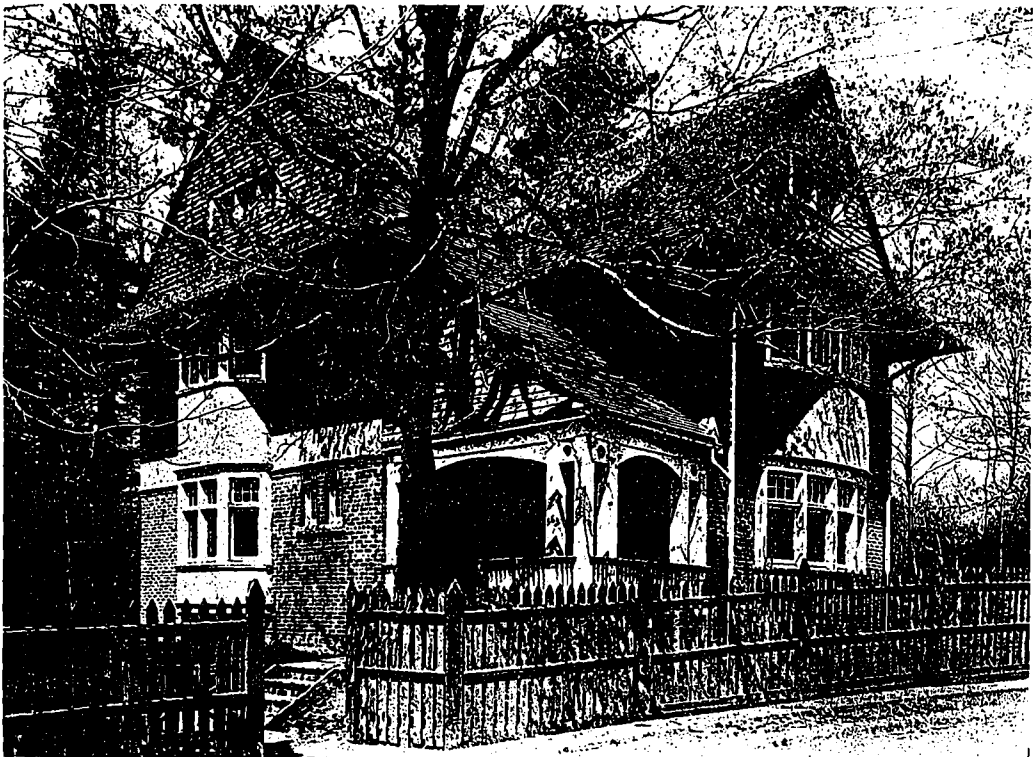
Villa Residence, 58 Popular Plains Road, Toronto. This House is Built of Red Brick for the Lower Portion, with Cement Plaster and Shingle Work Above. The Continuation of the Roof Over the Verandah is a Pleasing Feature, while the Picket Fence Across the Front is Exceedingly Appropriate to the Narrow Roadway with its Slow, Gradual Rise, which the House Overlooks. F. S. Baker, Architect.
