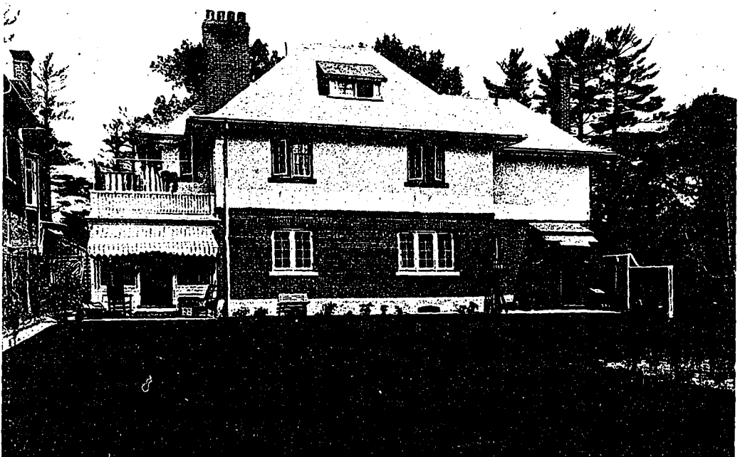
Rear View, Residence of Hugh S. Stevens, St. Clair Avenue, Toronto. John M. Lyle, Architect.
