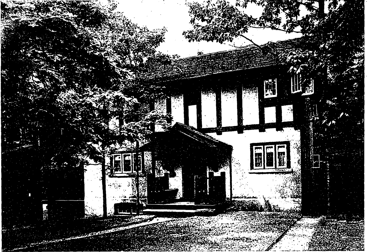
Residence of W. F. Temple, 106 Balsam Avenue, Toronto. An Attractive Small House Which Shows in an Interesting Manner the Use of Cement Stucco in External Construction. E. G. Wilson, Architect.
