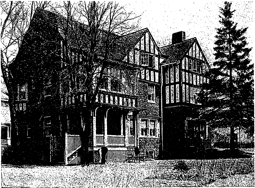
Residence of James Grand, 28 Oriole Road, Toronto. This Illustration Shows the Rear or South Elevation, on which Side all Main Rooms Have Been Placed. The Lower Story is of Extra Dark Red Brick, with White Mortar Joints while the Upper Story is of Half Timber and Stucco. Wickson and Gregg, Architects.
