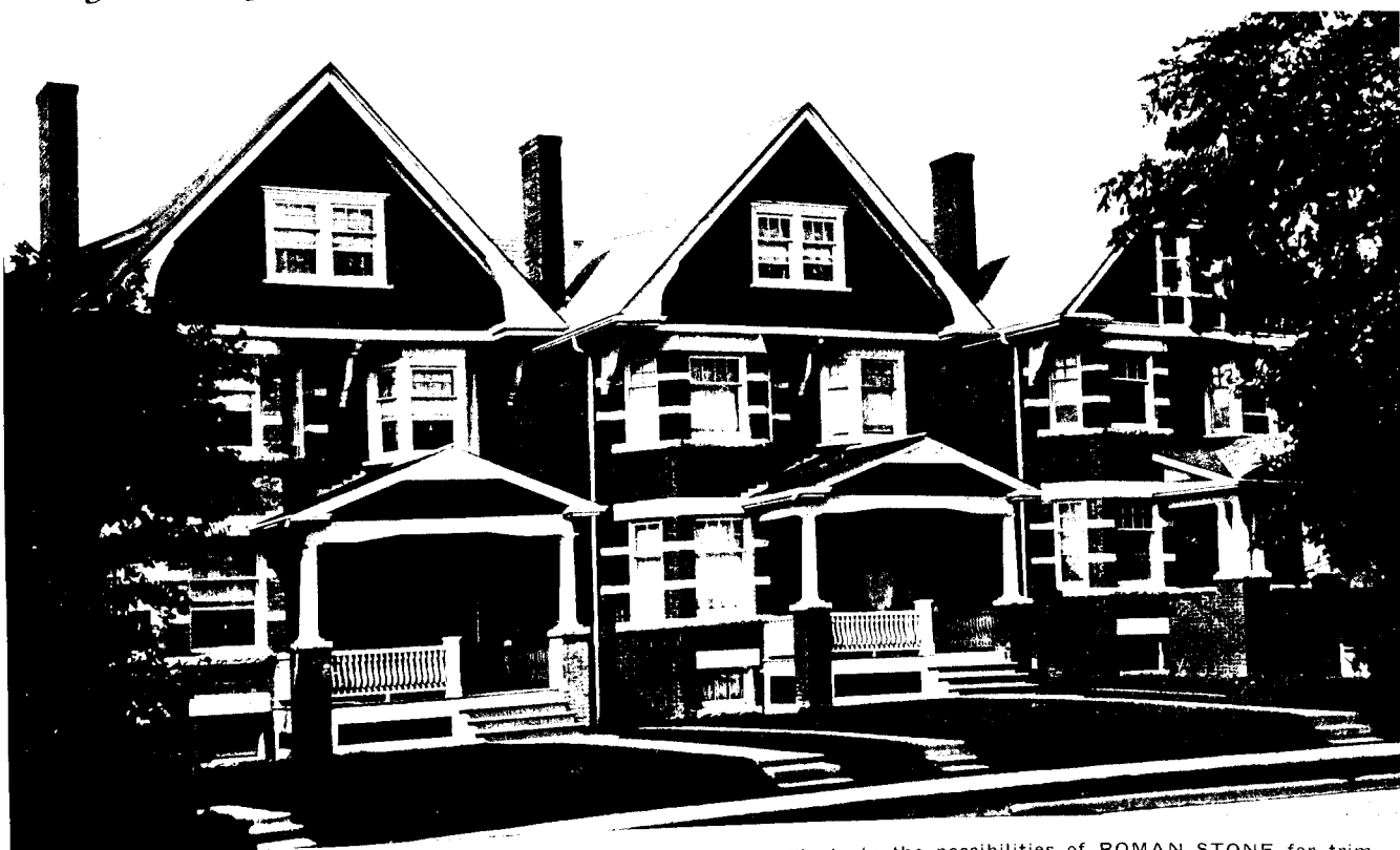
Dwellings, 276-278-280 Roncesvalles Avenue, Toronto. These buildings illustrate the possibilities of ROMAN STONE for trimmings on the moderate-priced dwelling.
