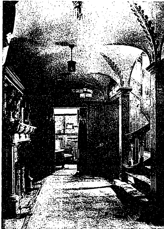
Lower Hall and Staircase, Residence of James S. Worts, Toronto, Finished in Quarter-cut Oak, with Panelled Dado of Same Wood. The Vaulted Ceiling is Embellished with a Stencil Decoration. Geo. W. Gouinlock, Architect.
