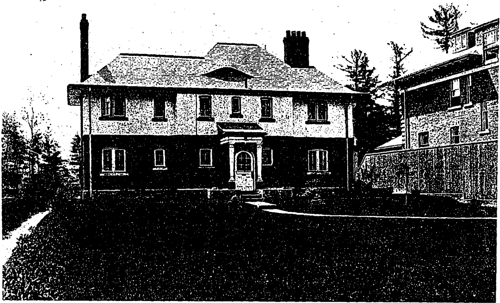
Front View, Residence of Hugh S. Stevens, St. Clair Avenue, Deer Park, Toronto. Though Simple in Character, the Poise of the Lines and Color Treatment of Walls and Roof Make the Design of this House Extremely Attractive. The Lower Storey is Built of Deep Red Brick with Wide Mortar Joints, and the Upper Portion is Treated with Greyish White Stucco on Brick, with a Roof of Grey Green Vermont Slate. John M. Lyle, Architect.
