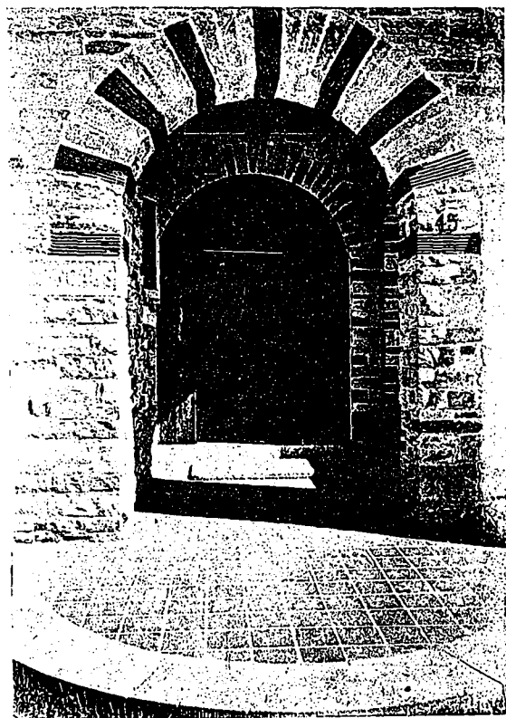
Entrance Porch, Residence of Charles H. Fleming, Castle Frank Crescent, Toronto. Note the Unusual Design of the Door, and the Unique Insetting of the Red Roof Tiles in the Stone Arches. Chadwick and Beckett, Architects.
