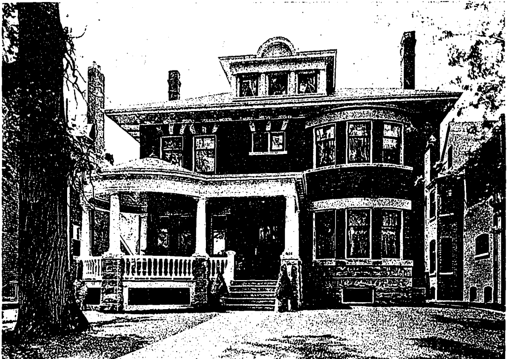
Home of H. Horseman, 185 Crescent Road, Toronto. A Residential Structure Designed along Modern Lines, with Red Brick Walls, Grey Stone Trimmings and White Painted Woodwork. Ellis & Connery, Architects.
