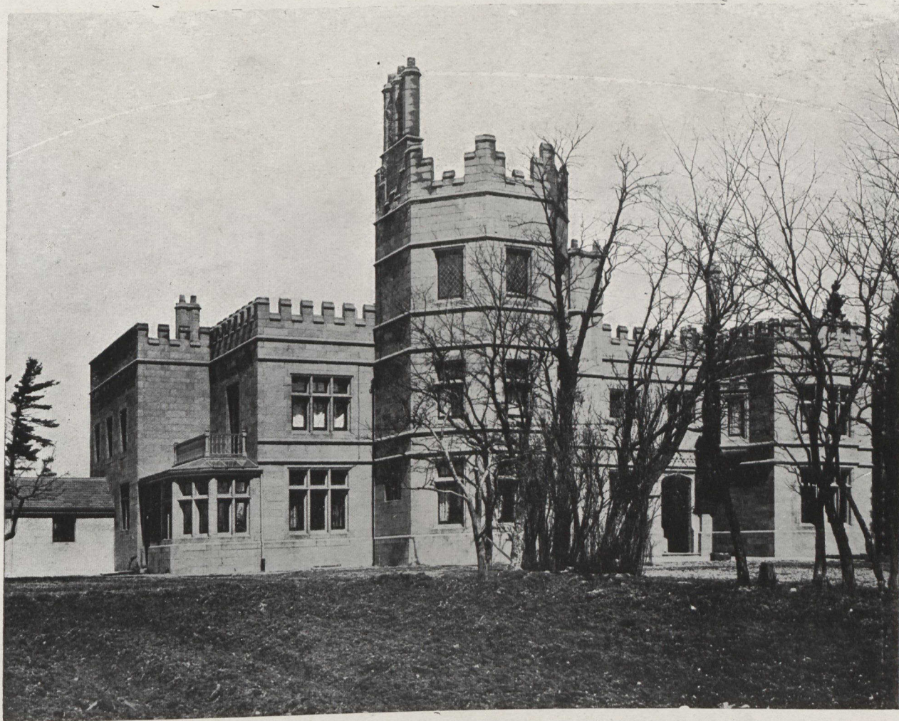
Residence of Mr. A. Ansley, at "Glen Grove," Eglinton. Geo. W. Guinlock, Architect.
