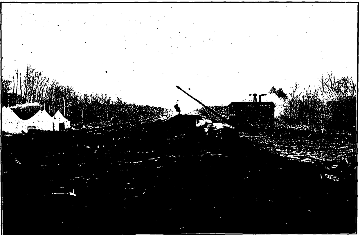
Grading G. T. P. Railway near Portage la Prairie.
