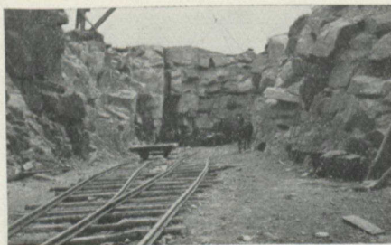
HEAVY ROCK WORK ON LAKE SUPERIOR BRANCH, GRAND TRUNK PACIFIC RAILWAY
