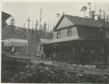
GRAND TRUNK PACIFIC TEMPORARY BUILDINGS AT PRINCE RUPERT
