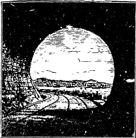
TUNNEL NEAR ST. BARTOLOMEO AND VIEW OF TRIESTE.
