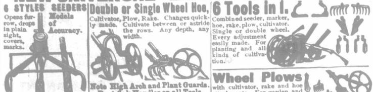
Opens furrow, drops in plain sight, covers, marks. Models of Accuracy. Cultivator, Plow, Rake. Changes quickly made. Cultivate between or astride the rows. Any depth, any width. Combined seeder, marker, hoe, rake, plow, cultivator. Single or double wheel. Every adjustment easily made. For planting and all kinds of cultivation.
