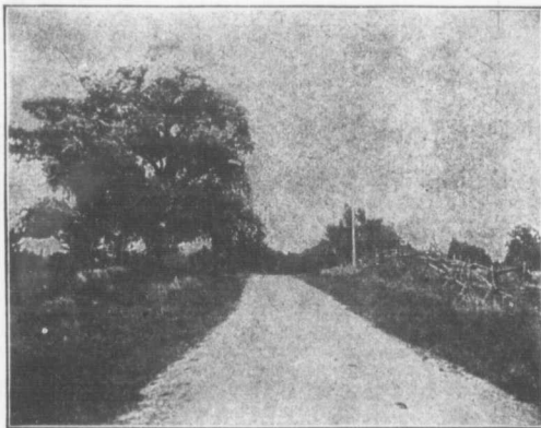
A Popular Piece of Good Road. Kerr Street, near Oakville, Ont. A tarvia filled macadam laid down in 1915. Photo after one year's service.
