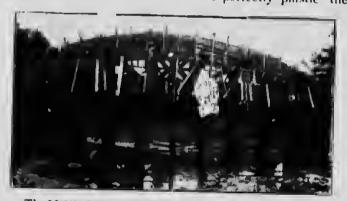
The Middle Road Truss Bridge, showing Forms in position
