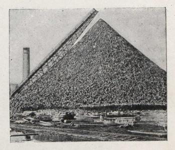
A travelling conveyor which is <sup>hoved</sup> on tracks along the face of the block pile is frequently <sup>used</sup> where wood is brought in on <sup>cars</sup> and in some cases also for <sup>blacking</sup> the wood on either side of the conveyor which carried the <sup>blocks</sup> to jt.
