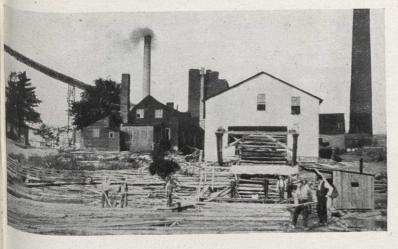
Log Hoist and Slasher House at the receiving end of a Pulp Wood Storage System.
