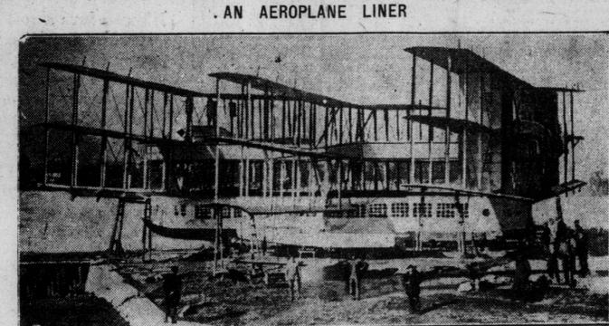
This, the latest invention of Signor Caproni, the famous Italian aeroplane designer, is capable of carrying 100 passengers. Its wings consist of three sets of triplanes with an area of 7,100 square feet. Eight engines developing 3,200 horse power propel it. Its total weight is 24 1/2 tons.
