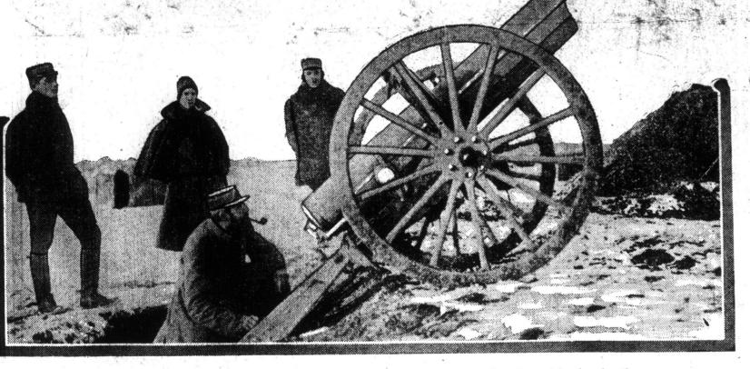
French artillery in action-Owing to the great elevation at which the gun is fired a pit must be dug for the gunners.
