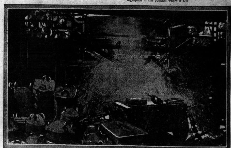
The question of munitions—The secret of the steel's strength; alloys being shot into the molten metal. A big circular furnace above the floor has been tapped, much as a barrel is tapped, and the molten metal has begun to flow into the 15 ton receptacle beneath, the alloys coming thru a shoot at the left, and mingling with the liquid steel.
