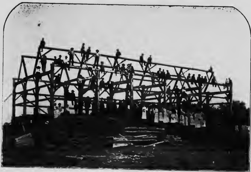
Barr Raking on Queenston. Cement concrete walls built by Messrs. John Sonley & Son London Ont
