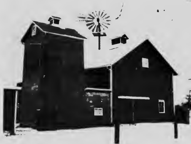
Quaker Concrete silo on farm of Mr. Jackson, Niagara-on-the-Lake, Ont.
