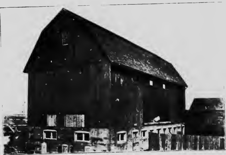
Another view of M. Vander... barn, showing end with ventilation pipe.
